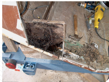
TOP: The rot was worse near the stringers, especially on the port side.
